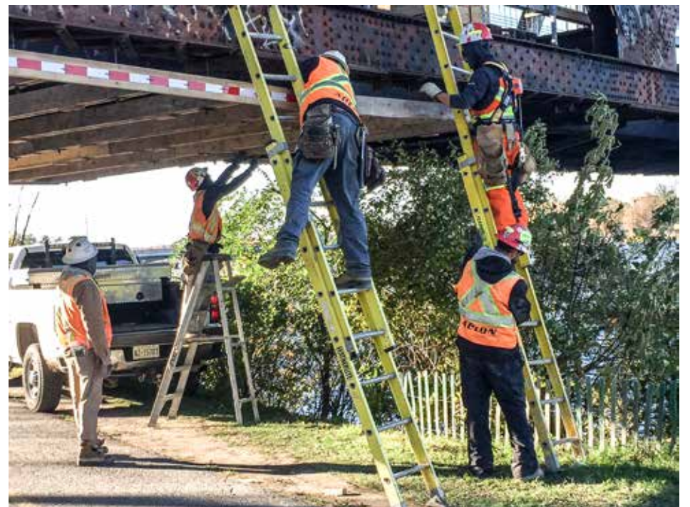
Crews started work on the Commanda bridge in 2021.
