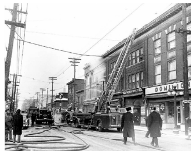
The site of the proposed development after its 1950 fire. The buildings have been little altered in the intervening years.
