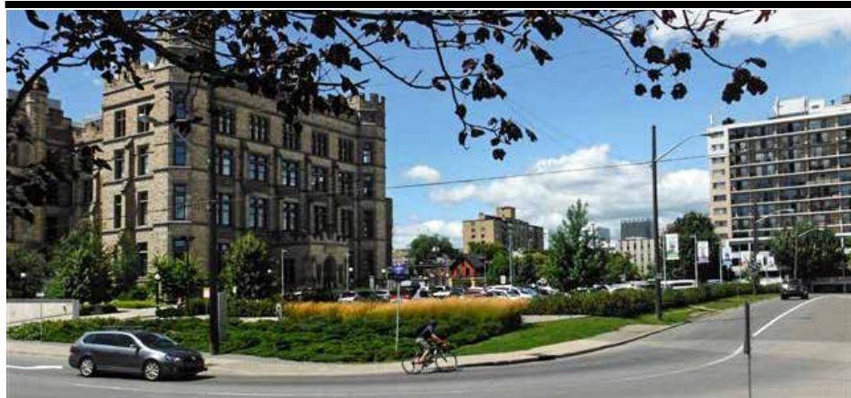
A new sidewalk is to be added on Metcalfe from Argyle to McLeod.
