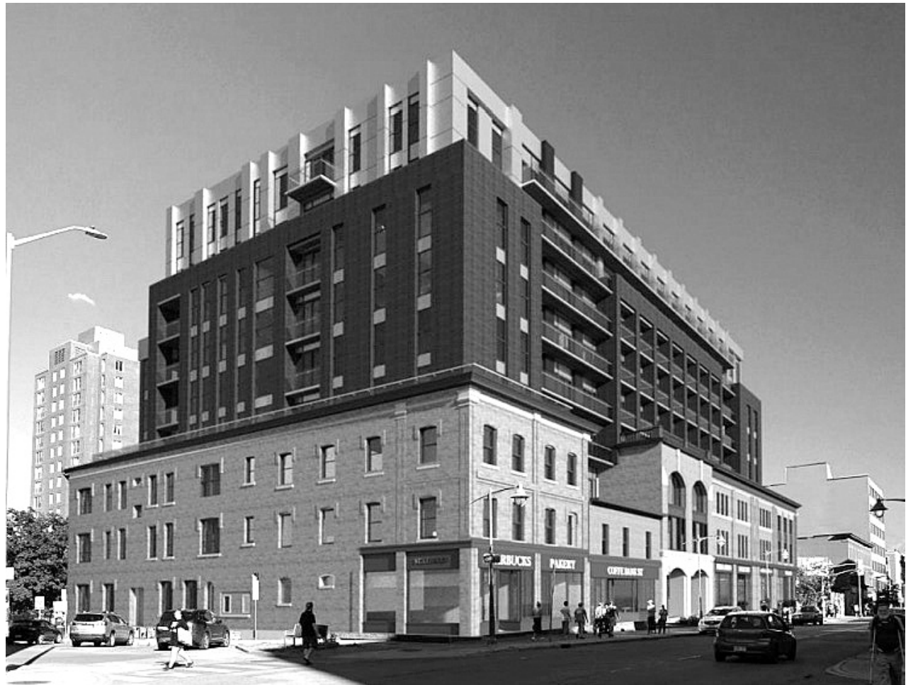
This full block on Bank from Nepean to Lisgar Streets may receive a major addition on top. A skilful blending of new and old?
