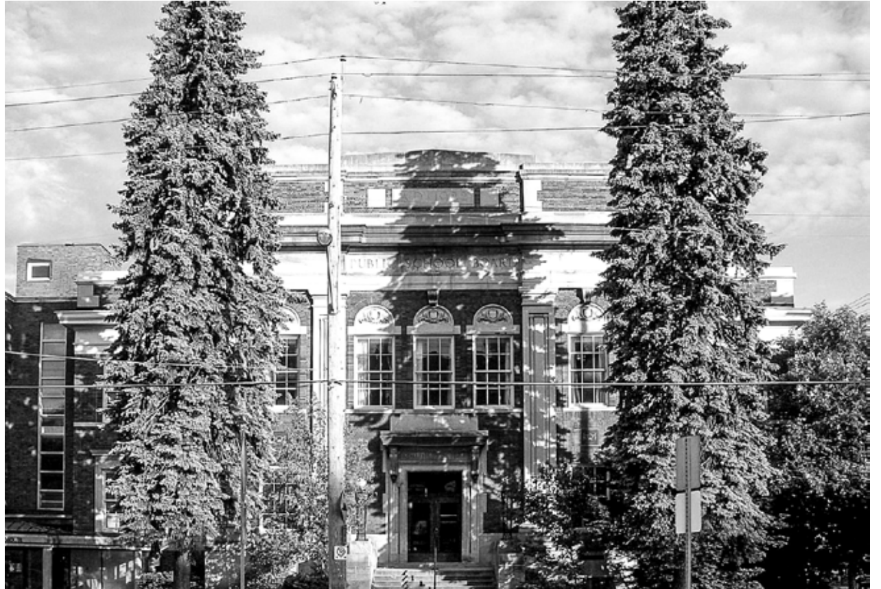
The former Ottawa Board of Education headquarters on Gilmour Street, now owned by Ashcroft Homes, has been vacant for over 20 years. Serious wall and foundation settlement is now occurring. It has recently been boarded up in an effort to prevent further water penetration.
