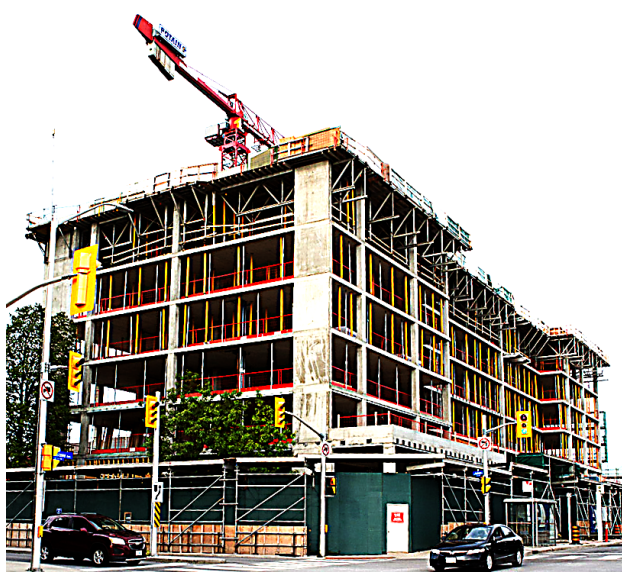
811 Gladstone under construction.
